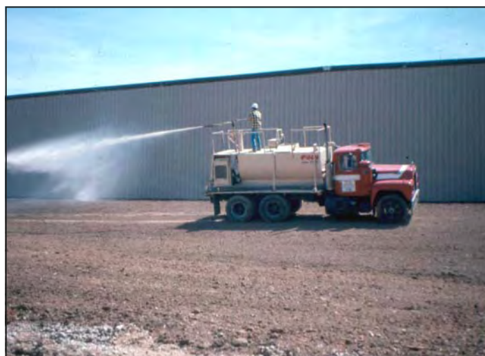
Figure 3: Hydroseeding
