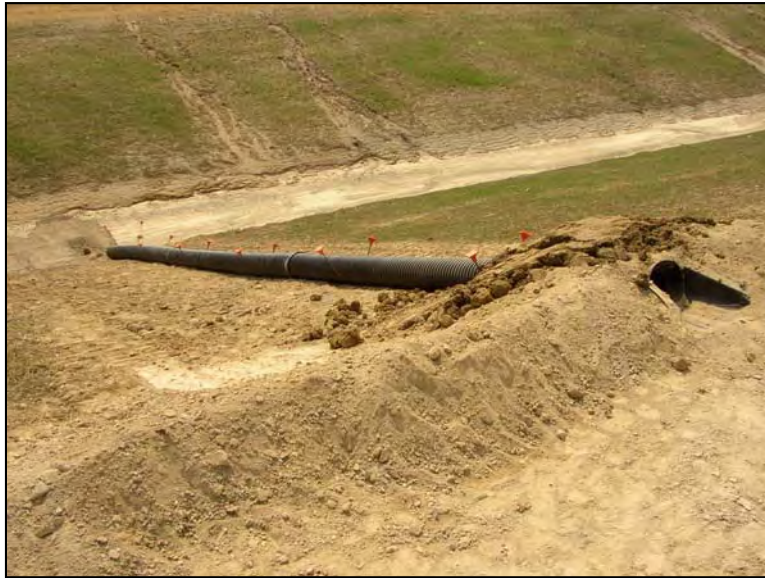
Figure 1: Temporary Slope Drain with Flared-End Section
