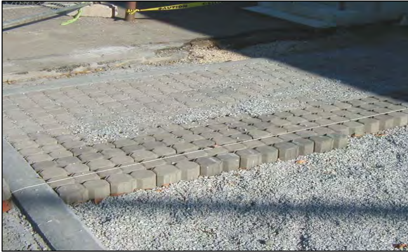
Figure 1: Installation of a Permeable Paving System
