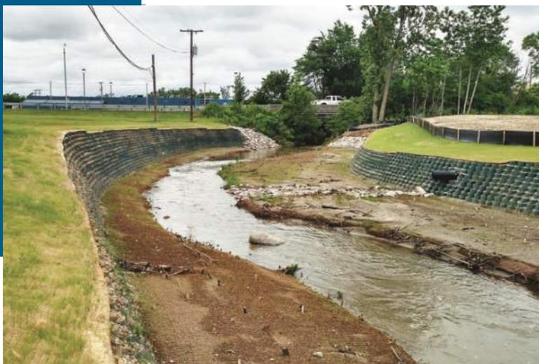
Upon completion of the installation of the cellular confinement system in 2015, Fort Wayne experienced one of the wettest summers on record. While a large portion of the city experienced flooding, the two-stage channel and confinement system was inundated but withstood its first test.
