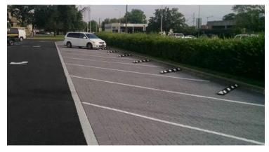
project was designed with an infiltration bed installed under the parking lot to redirect over two million gallons of rain water annually away from the combined sewer system. The result of this design was an agreement with EWSU to contribute \$414,742 to the construction of the project, representing a considerable financial incentive for the developer.
