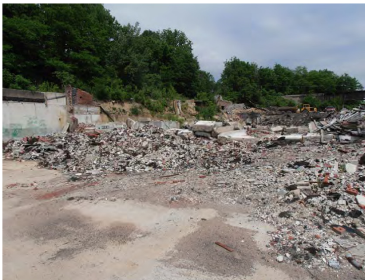
Picture 6. Brick and concrete pile, looking northwest.
