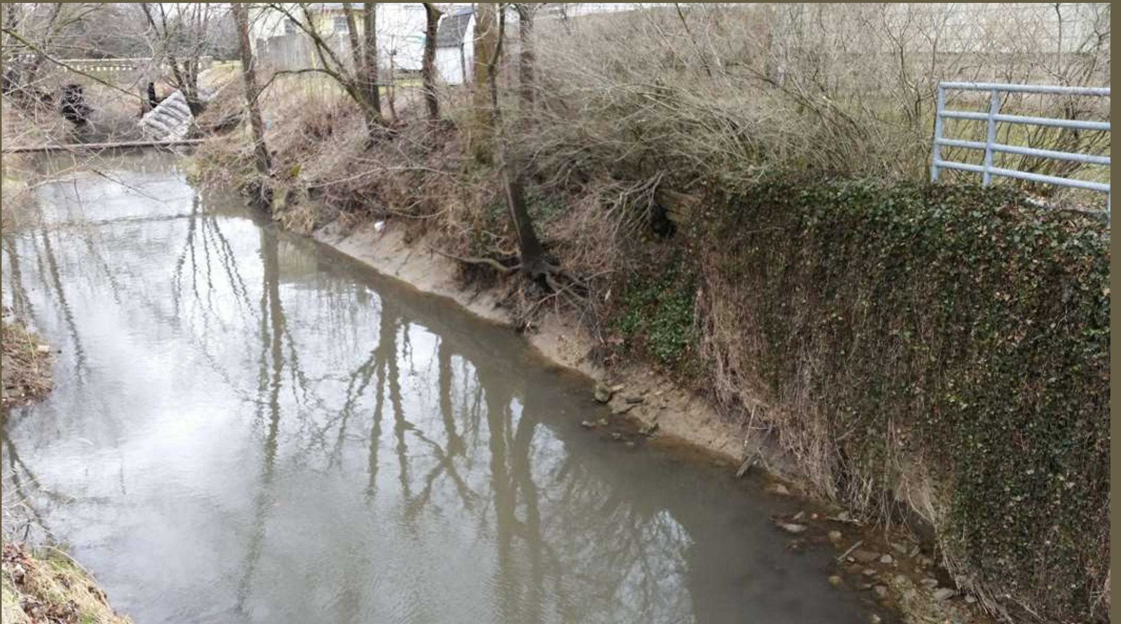
Left bank looking upstream from the Meridian Street Bridge. The scour line is visible along the left bank. Note the gabion baskets at the upstream end.
