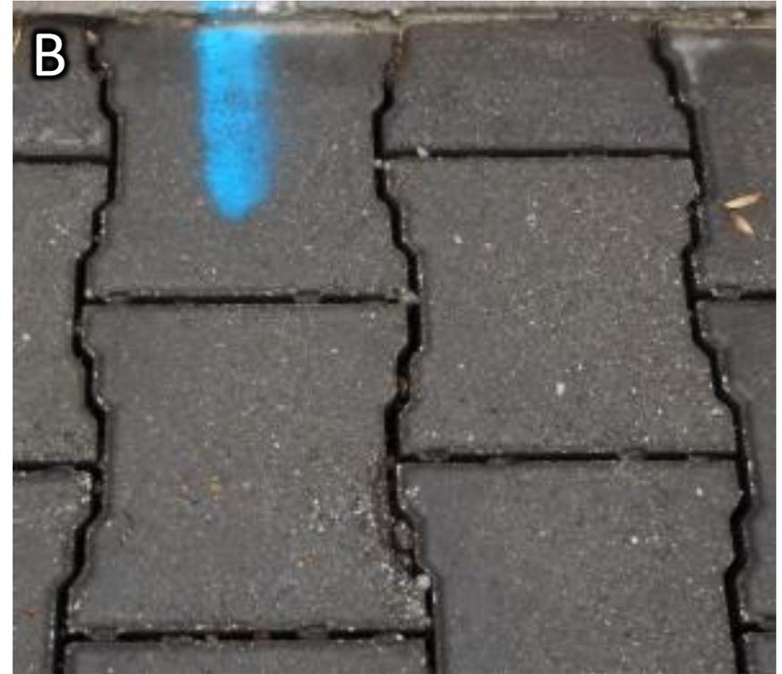
**Permeable articulated concrete blocks/mats before (A) and after (B) cleaning with a Vac Head.**
