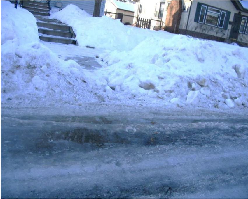
**Slush gathering and refreezing on the traditional asphalt at Site 1 on January 17, 2010**
