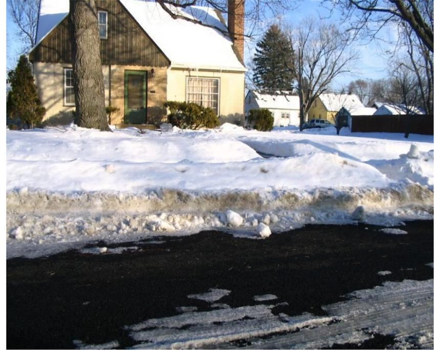
**Slush free porous asphalt on January 17, 2010**
