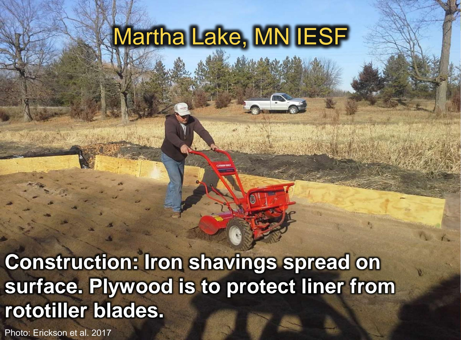
**Construction: Iron shavings spread on surface. Plywood is to protect liner from rototiller blades.**
