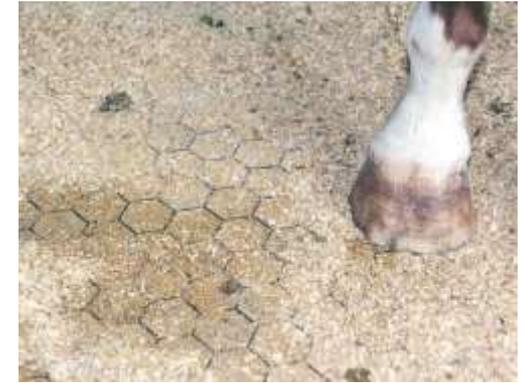
**Porous pavers** are manufactured in a variety of designs and materials. Concrete turfblock for grass paving began in the mid-1940's and plastic versions were invented in the late 70's and early 80's. Porous pavers are generally a cellular grid system filled with dirt, sand, or gravel.
