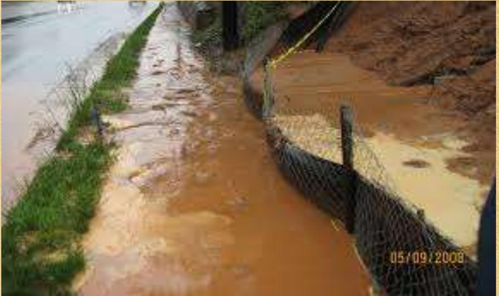
Added Wire Backing, Increased Stake Spacing and Size?
