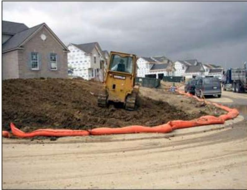
*A filter tube/filter sock is a temporary barrier consisting of permeable material (i.e., aggregate, compost, excelsior, or straw, etc.) contained in a permeable geotextile fabric or non-biodegradable net matrix installed to intercept and treat sediment-laden runoff from small, unvegetated drainage areas.*
