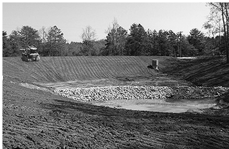
Retention Pond Under Construction
