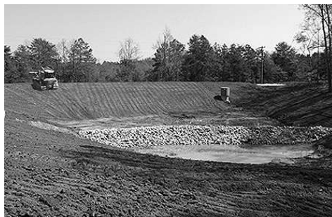
Retention Pond Under Construction
